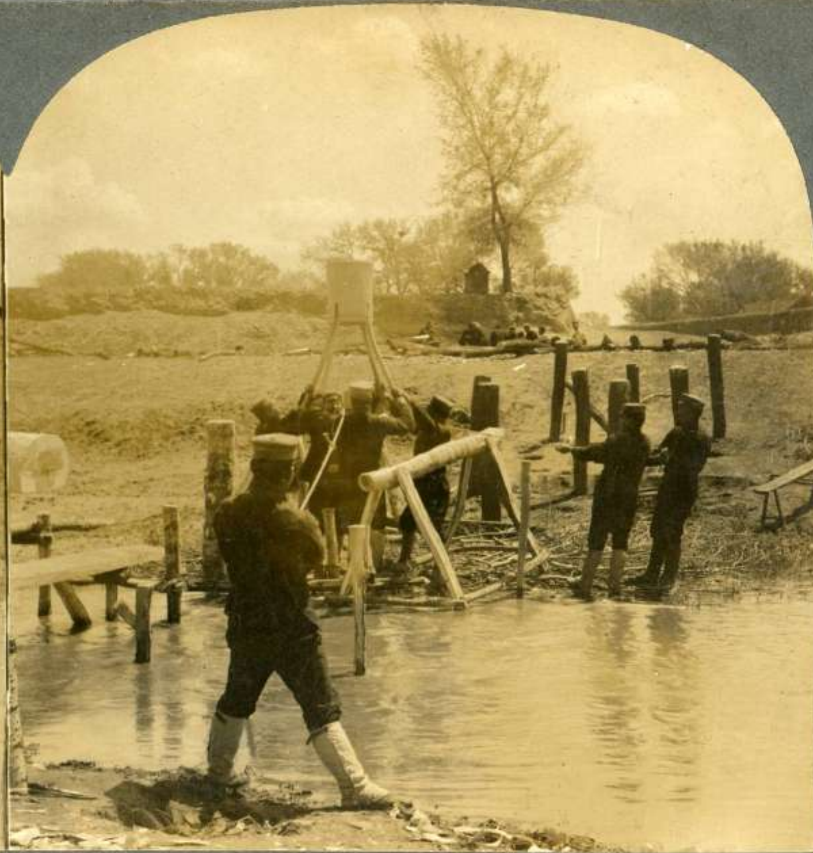
6598—Japanese Bridge Engineers Driving Piles by Hand Power, Manchuria.
