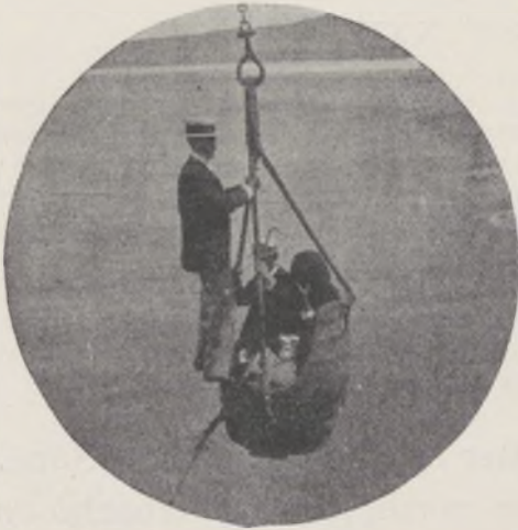
LANDING BY MEANS OF TUB, SALAVERRY.
