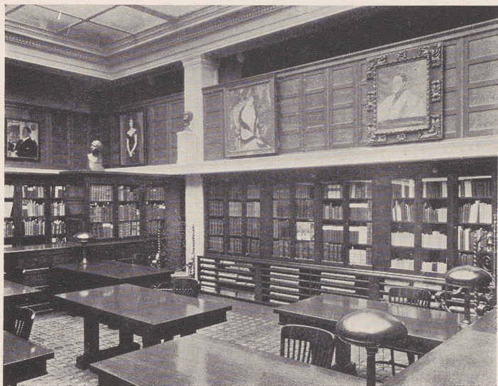
VIEW OF READING ROOM
