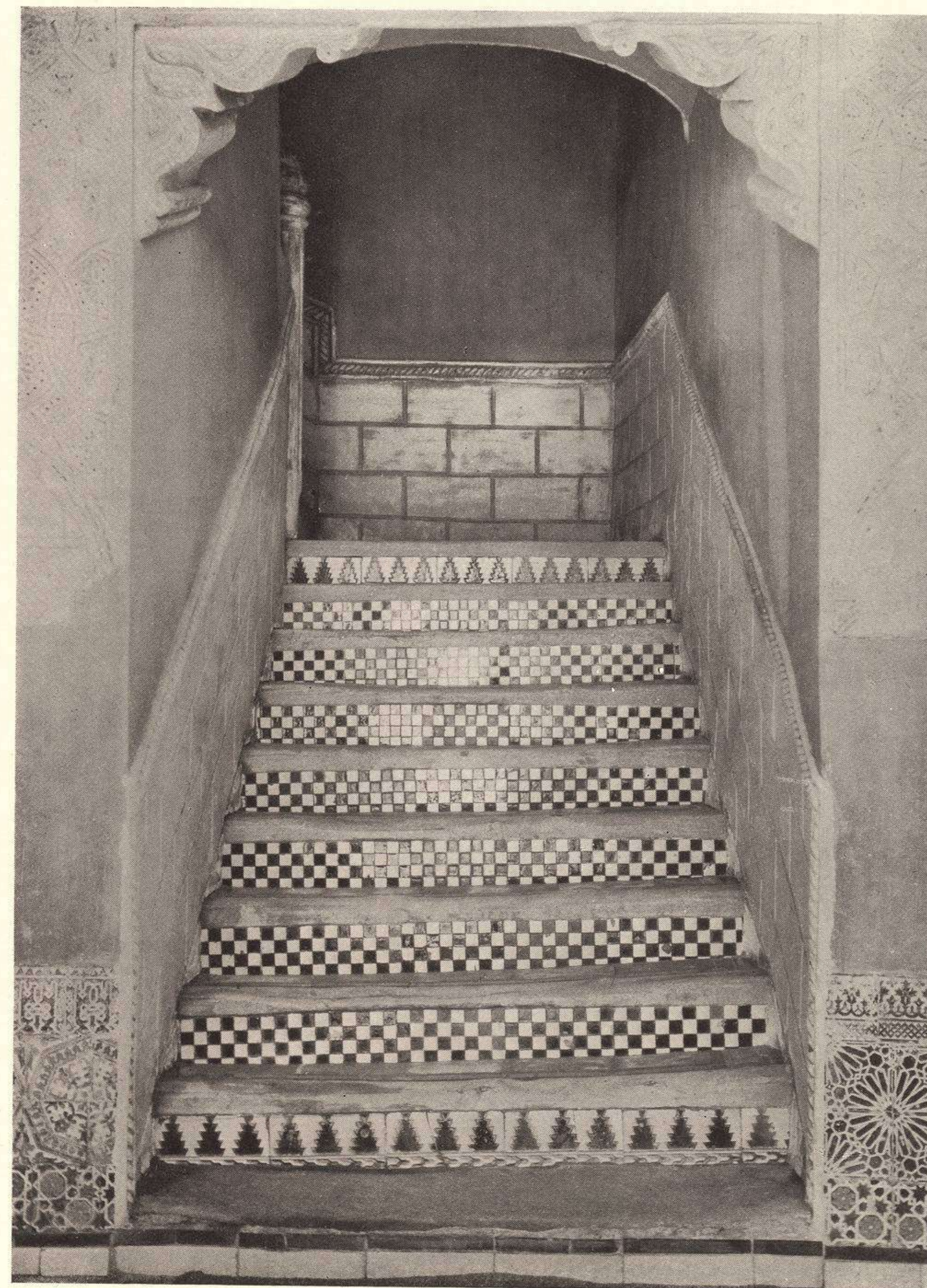
TOLEDO, HOUSE OF EL GRECO. STAIR LEADING UP FROM PATIO; RED TILE TREADS, POLYCHROME TILE RISERS, WOODEN NOSING
