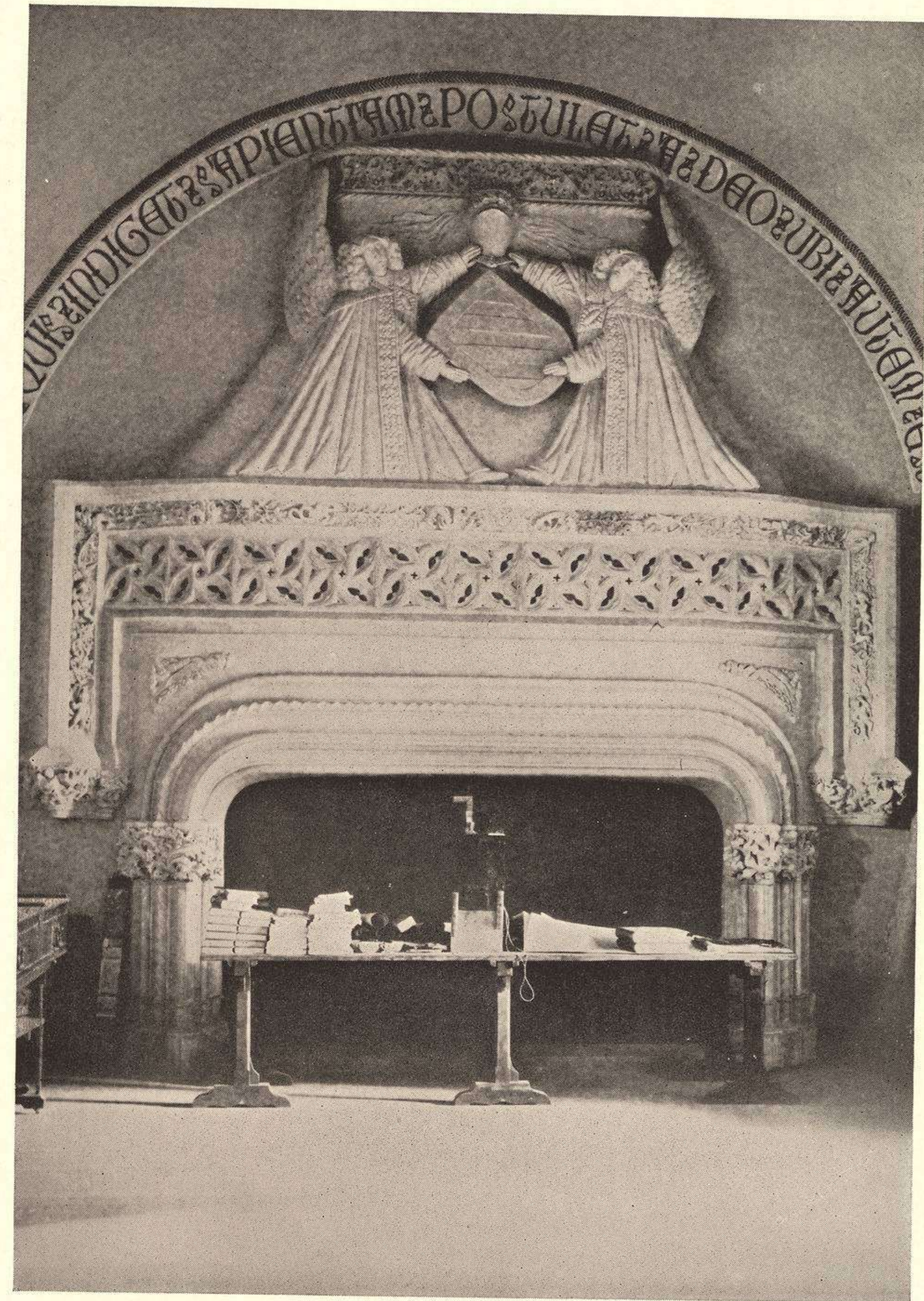
GUADAMUR, CASTLE OF THE CONDE DEL ASALTO. THE GREAT STONE CHIMNEY-PIECE IN THE HALL, WITH OPENING OF NINE FEET. THE FRIEZE OVERHEAD IS INSCRIBED IN BLUE ON A WHITE BACKGROUND
