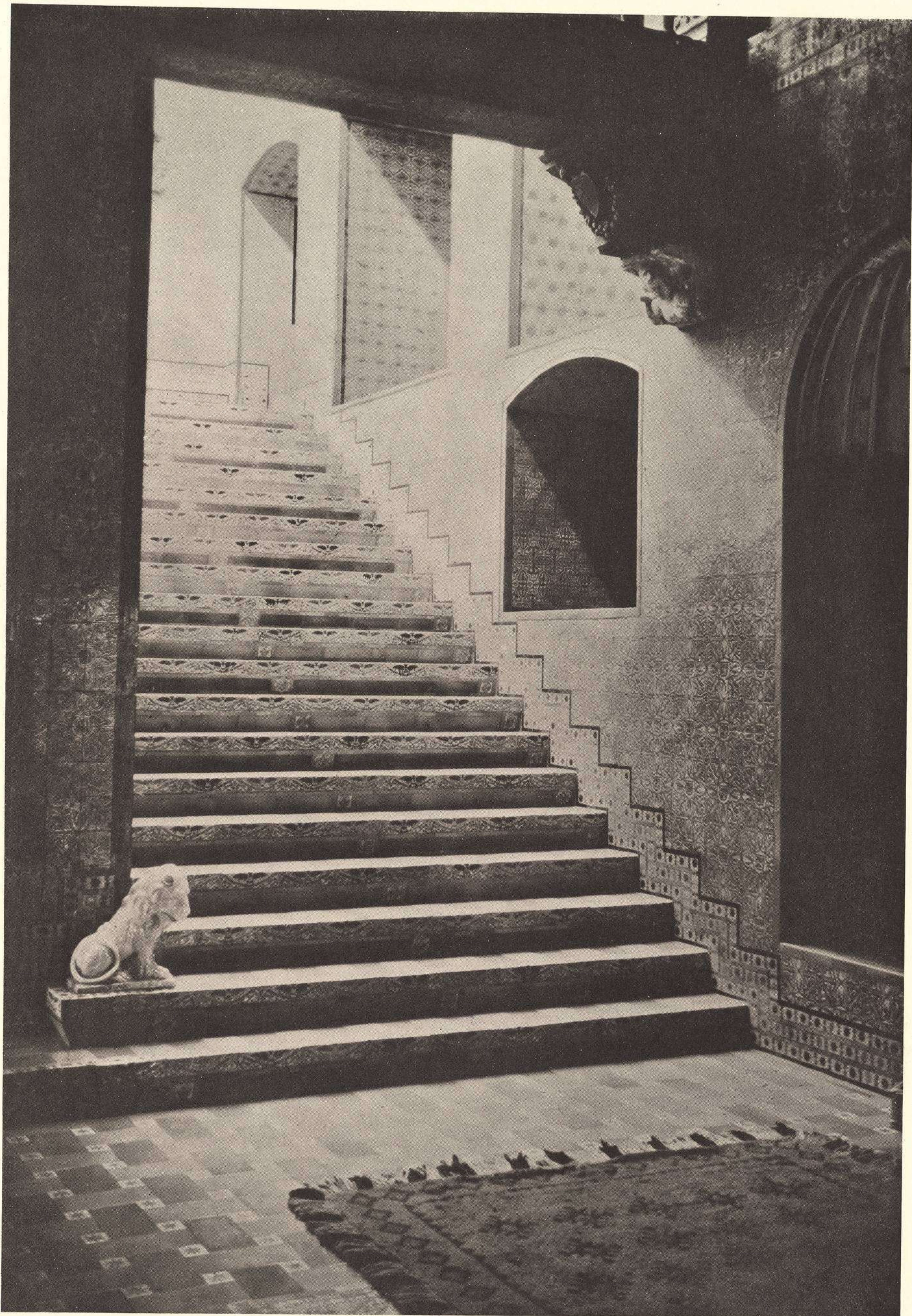
SEVILLE, PALACE OF DON MIGUEL SANCHEZ-DALP. MAIN STAIRWAY TREATED IN POLYCHROME TILES AND SGRAFFITO
