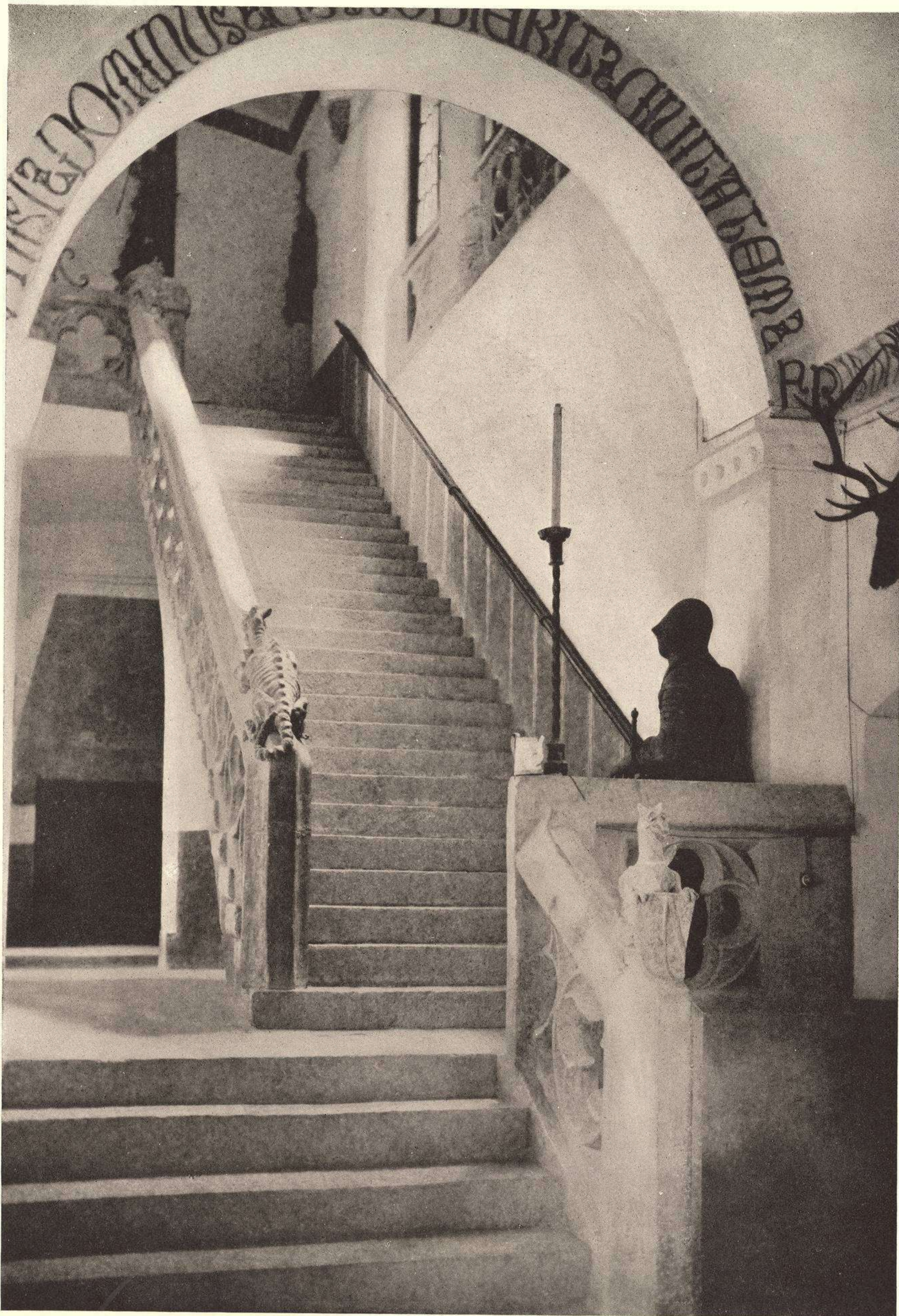
GUADAMUR CASTLE, XV CENTURY GRANITE STAIRWAY. LETTERED FRIEZE IN BLUE AND WHITE FOLLOWING THE MOORISH TRADITION COMMON THROUGHOUT THE PROVINCE OF TOLEDO
