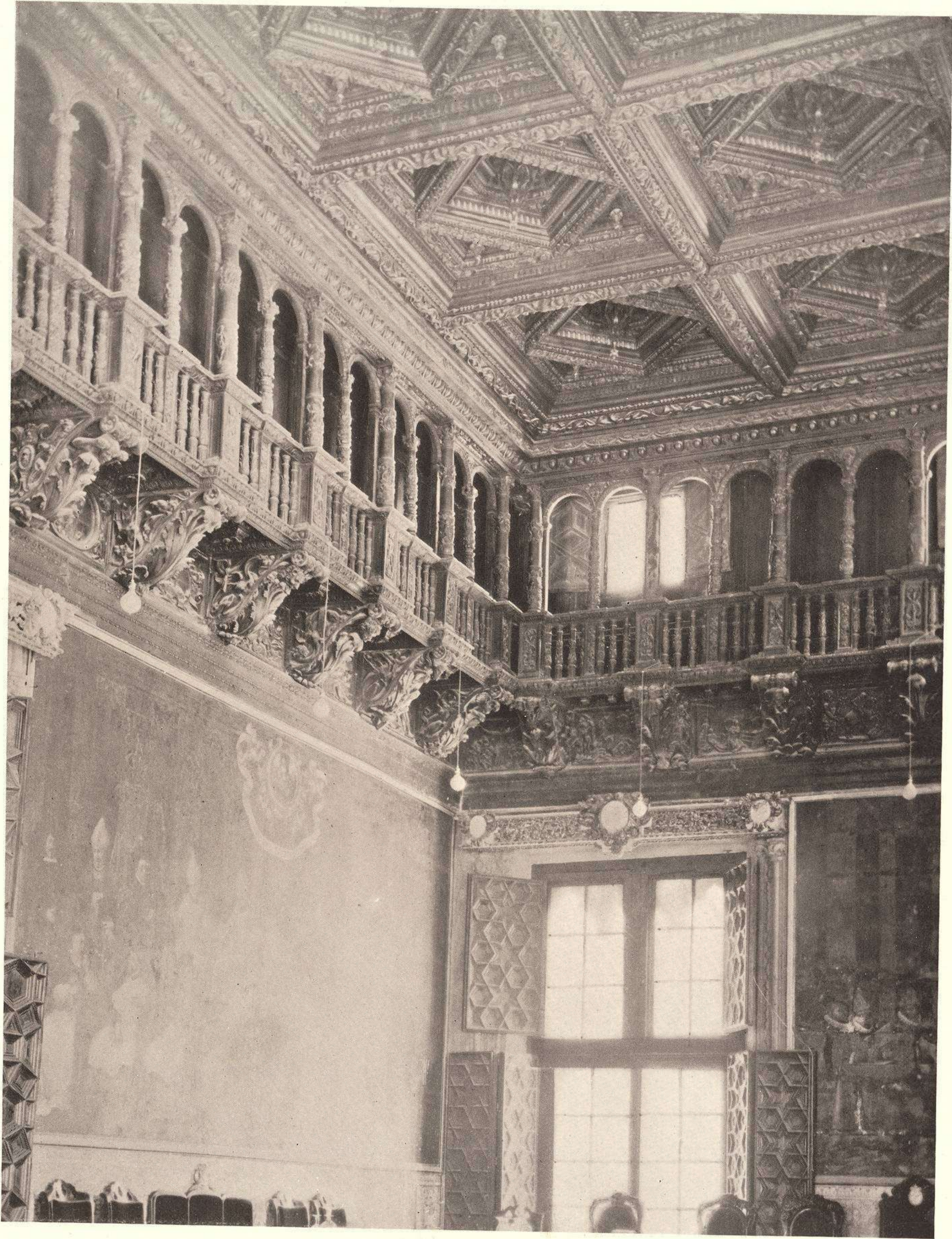
VALENCIA, THE LAW COURTS, OR AUDIENCIA. SUMPTUOUS XVI CENTURY SALON WITH COFFERED CEILING AND OPEN GALLERY OF CEDARWOOD UNDECORATED; WALLS PAINTED IN FRESCOES ABOVE A WAINSCOT OF POLYCHROME TILES; SHUTTERS OF MOORISH CARPENTRY
