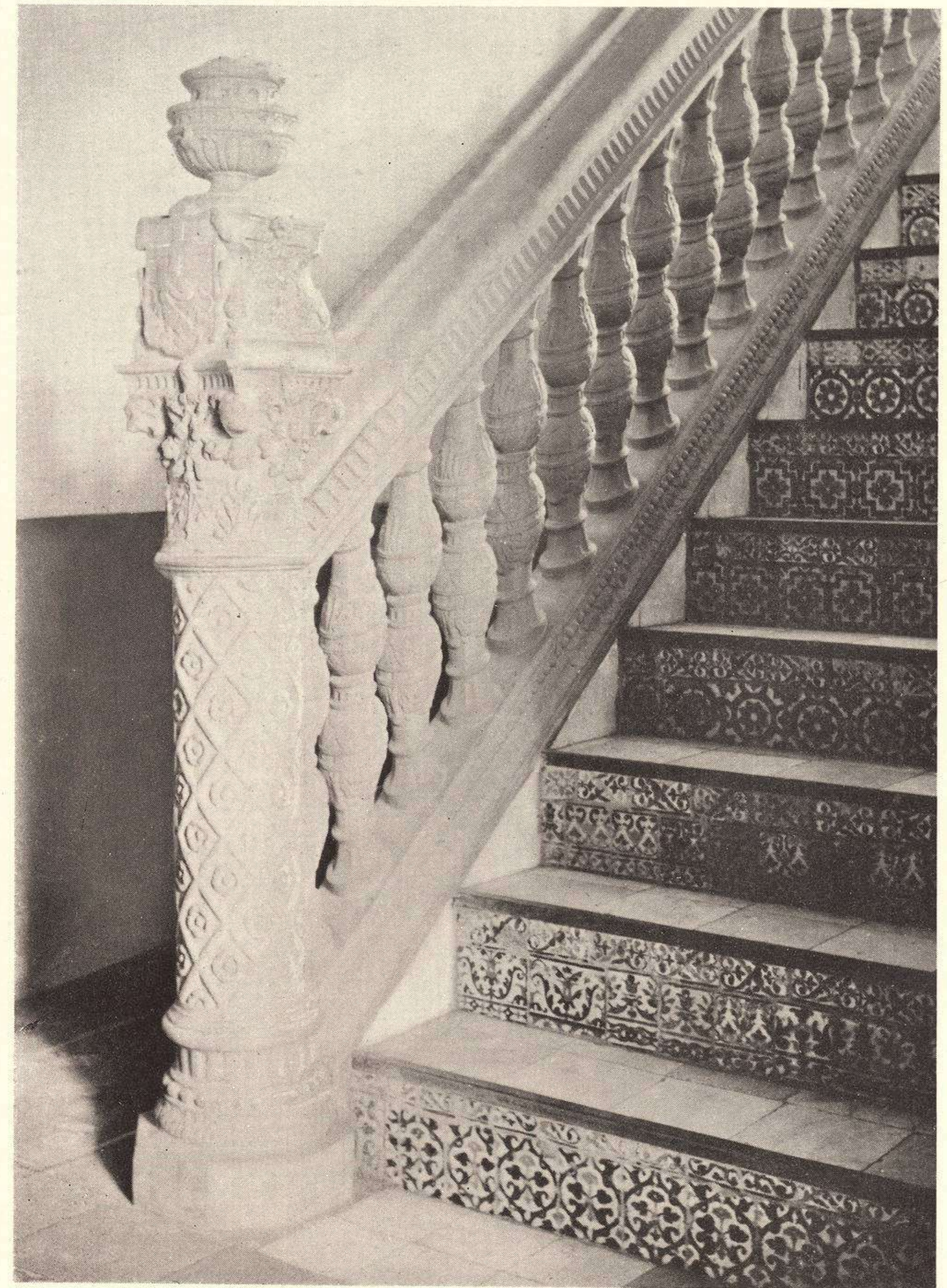
TOLEDO, HOUSE OF THE CONDE DE TOLEDO. STAIR OF POLYCHROME TILES AND STONE
