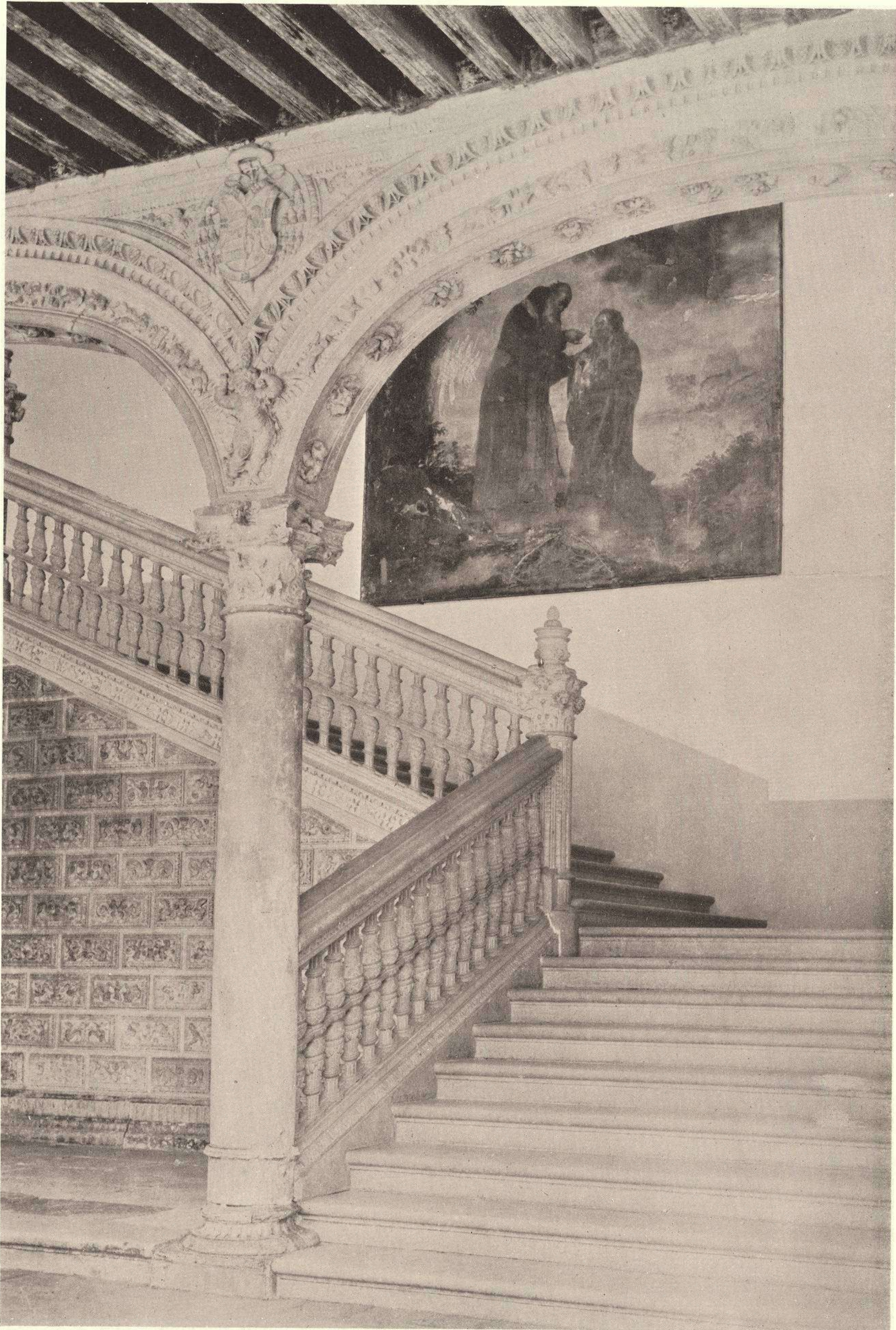
ALCALA DE HENARES, EPISCOPAL PALACE (MIDDLE XVI CENTURY). GRAND STAIR OF THE PATIO, CARVED IN YELLOWISH MARBLE; WOODEN CEILING DECORATED IN COLOR
