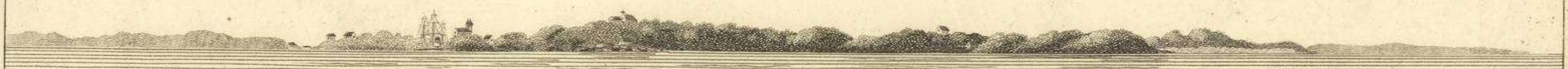
View of the entrance of the Harbour
