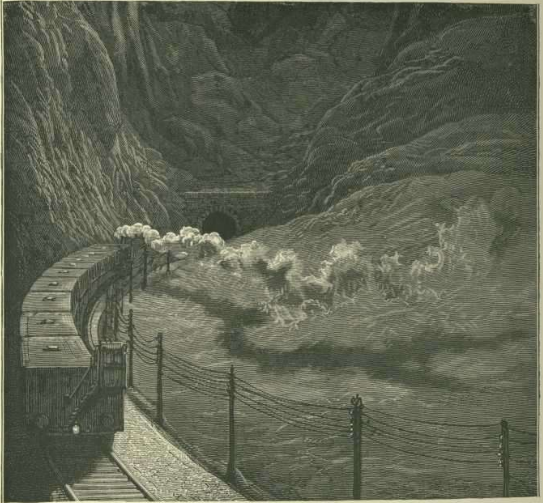
GORGES OF FANCORDO : THE TUNNEL.
