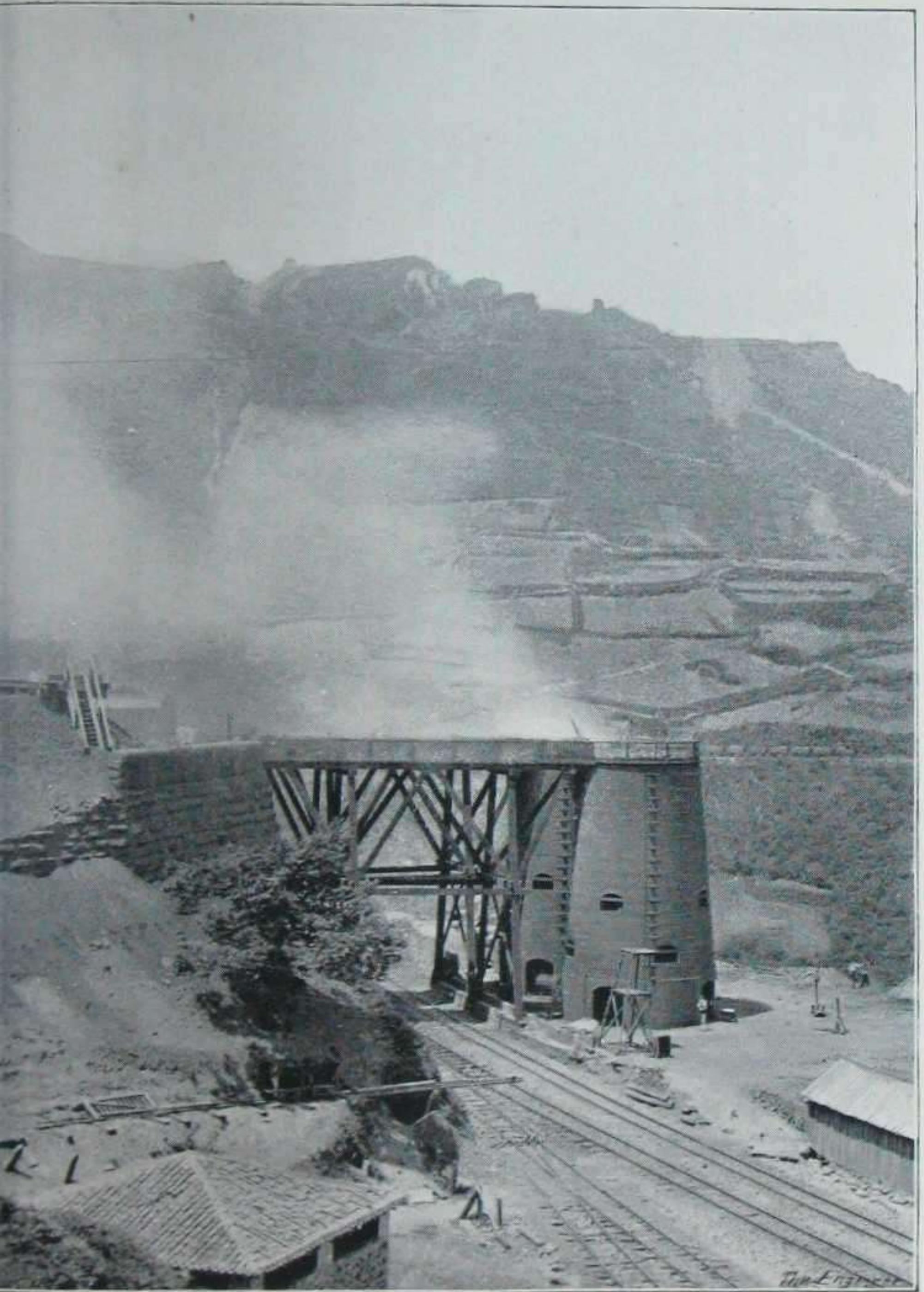
Calcining Plant for Spathic Ore. Orconera Company.
